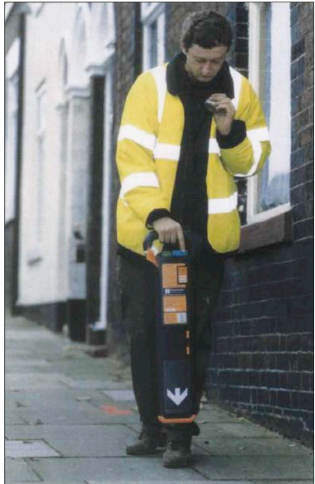
Figure 5 Using a cable locator
