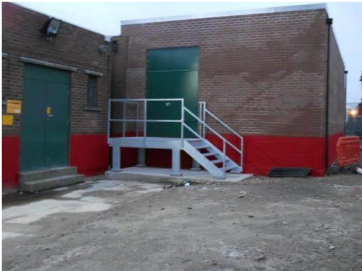
Raised building floor with step access. (Courtesy WPD)
