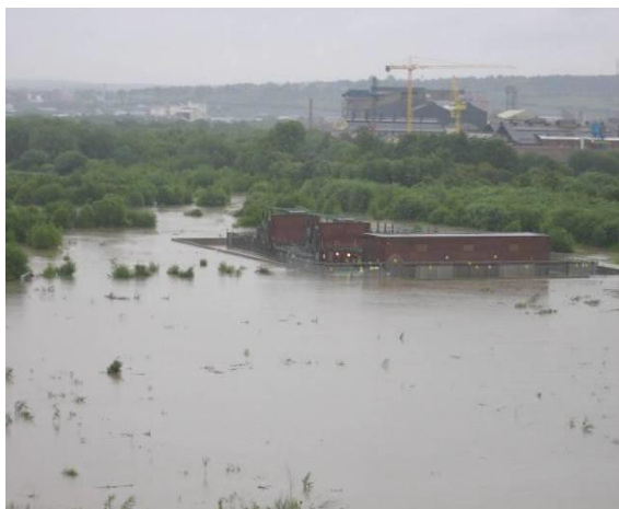
An electricity substation protected by flood barriers in the 2007 floods in the North East of England
