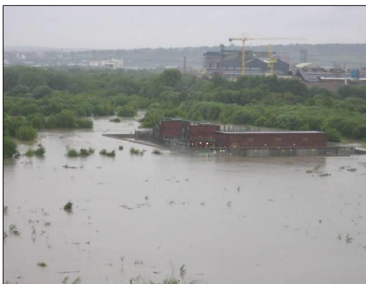
Photograph 1 - An electricity substation protected by flood barriers in the 2007 floods in the North East of England
